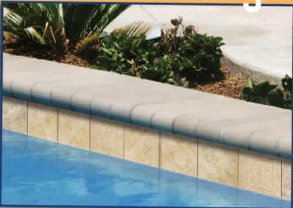
Tile shown in photo above is Bellagio BEL-6BLEND Beige and BEL-DECO Beige.
