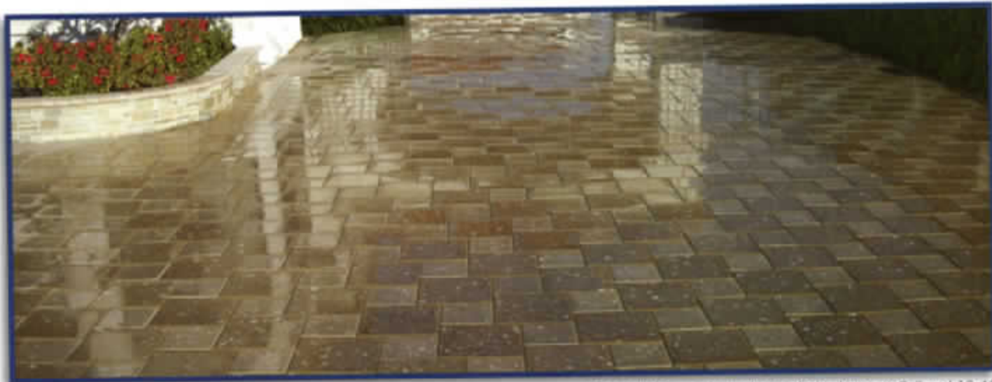
Roadlock Pavers shown in the photo above are 8x8 and 12x12 Artistic Pavers Shellock Cappuccino and Desert Series Sand.
