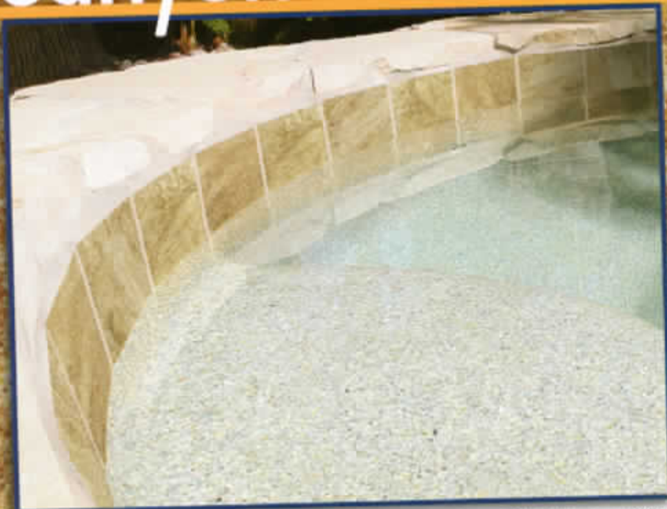
Tile shown in photo above is Canyon Stone Tan CNS-TAN6 and StoneScapes Tahoe Blue aggregate finish.
