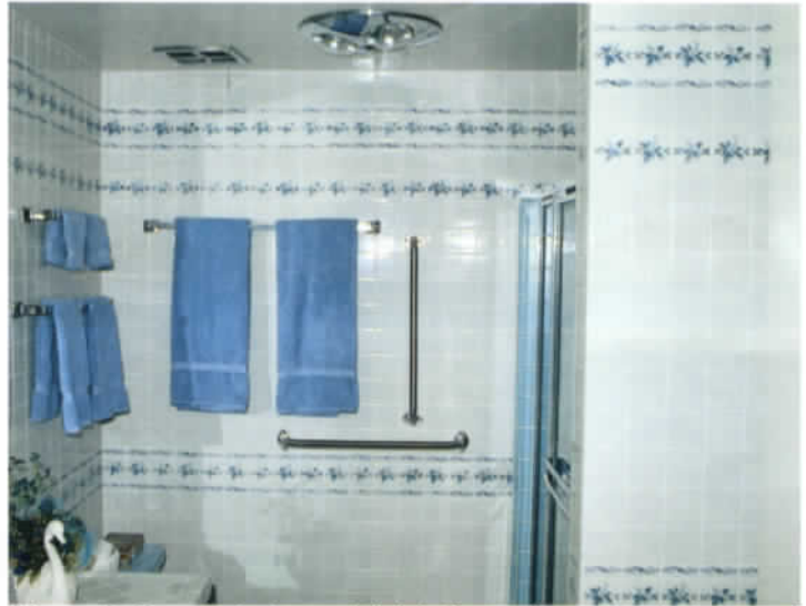
Almond Monet Autumn Field tiles with multiple rows of Almond Monet Autumn. Beauty and ease of cleaning were both achieved by installing tile floor to ceiling.
