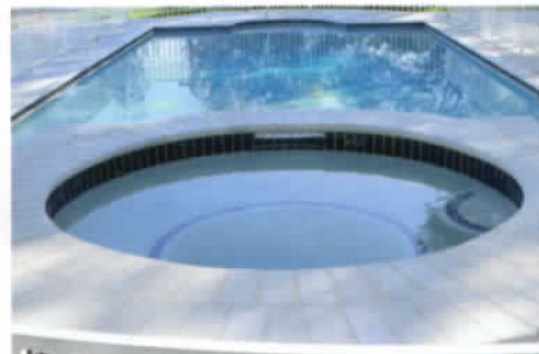
Top 2 photos show a pool & spa with White Bullnose Brick Coping on the spa & steps. White Bullnose Coping frames the pool. 2x6 Cobalt Blue tile on pool & spa.
