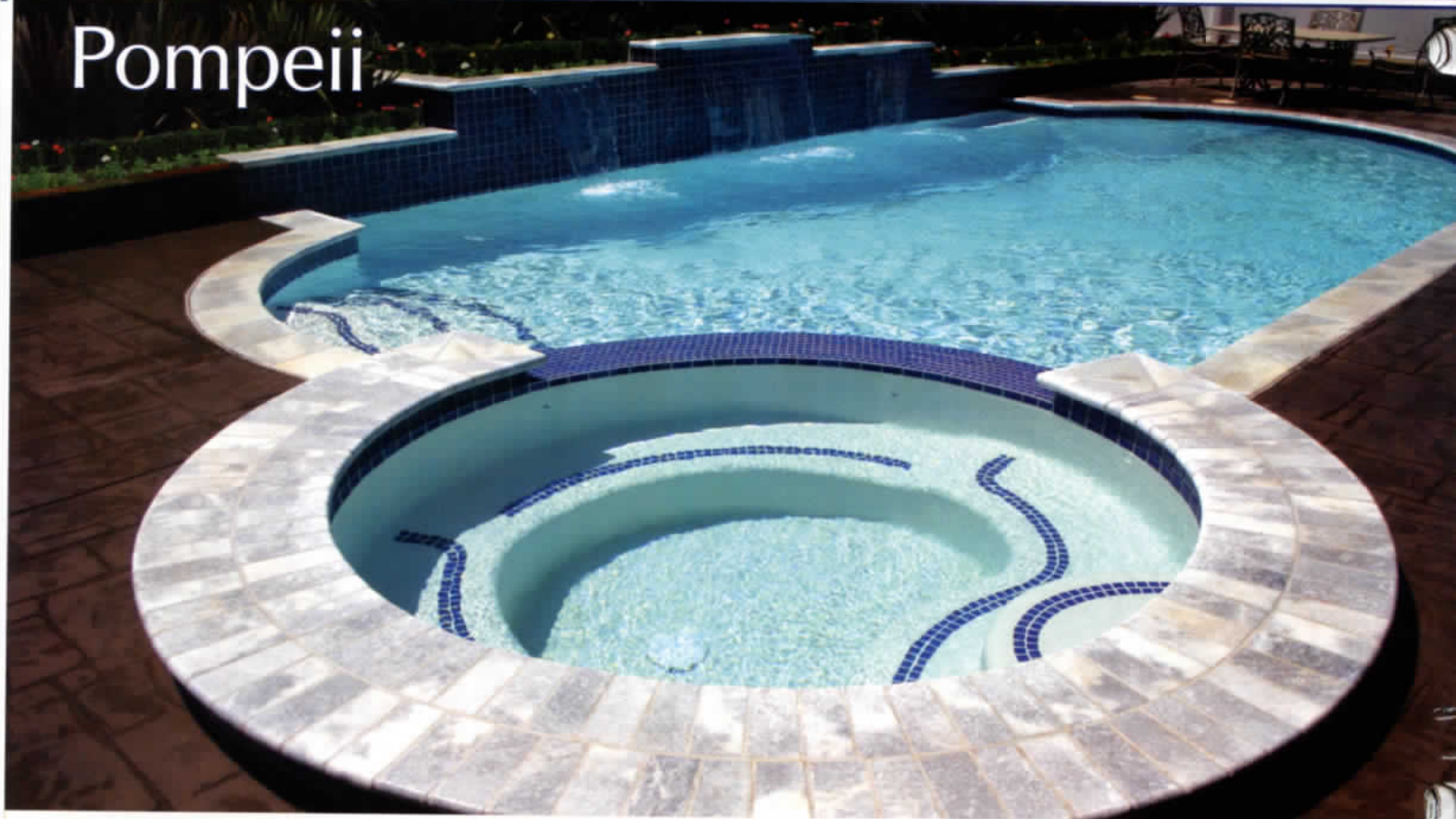
Pool Waterline: Pompeii Steel Blue 3" x 3". Raised Wall: Pompeii Steel Blue 3" x 3" & Steel Blue Deco 6" x 6". Spa Stairs & Spillway: Pompeii Steel Blue 1" x 1", Coping: Marmore Stone Branco 4" x 12".
