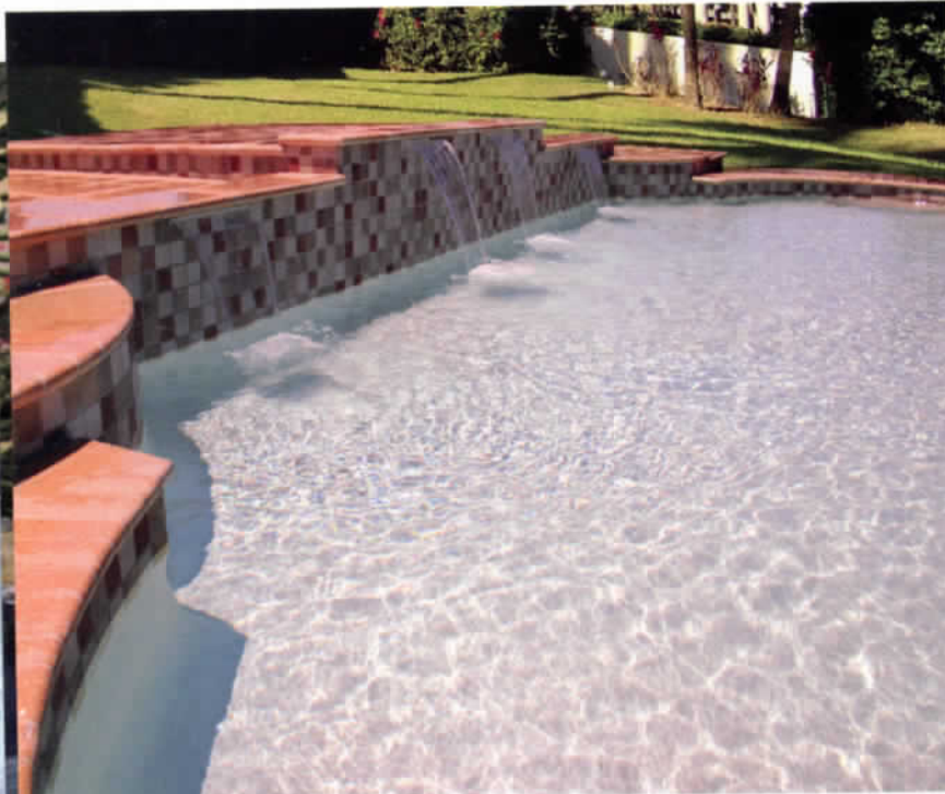
Pool Waterline & Raised Wall: Vintage Mosaic Mix 3" x 3".
